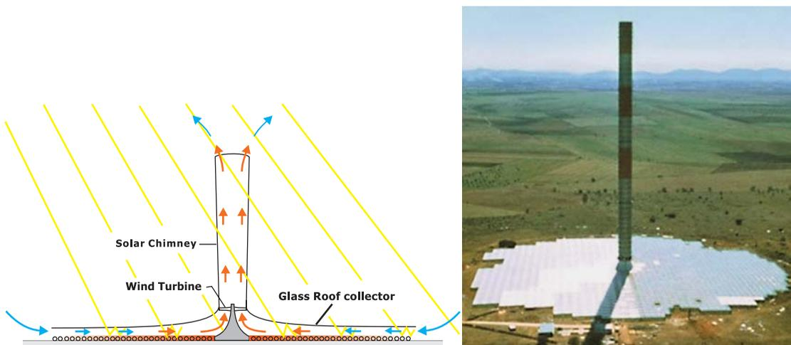
**Figure No. 6 Principle and Prototype of the 195 m high solar chimney (50kW power plant) at Manzanares, Spain, which was in operation between 1982 and 1989.**
